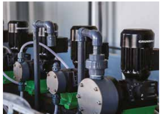
Consumables dosing pumps
