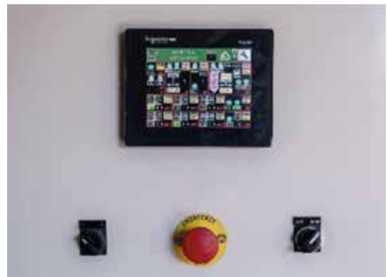
Typical control panel of a ZEOLAGIC installation
